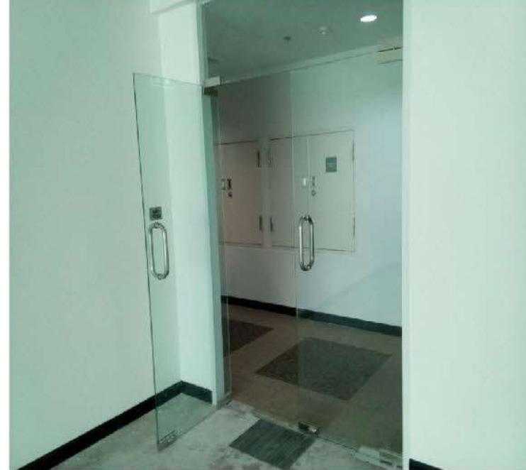
Glass Door Entrance : Double door with door handle and keys (Building Standard)
